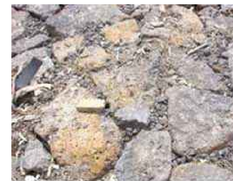
EXAMPLE OF WELL INTERLOCKED ROCKWORK WITH SEALED VOIDS
